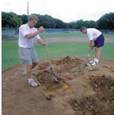
STEP 2: Cut out and remove all loose dirt from the high stress area surrounding the pitcher's mound to a depth of 3".
