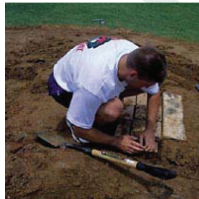
STEP 3: Place Diamond Pro® Mound / Home Plate Clay Bricks as evenly and close together as possible.
