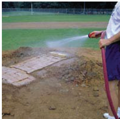
STEP 4: Once the bricks have been placed, water the cut area. Tamp the bricks into place.
